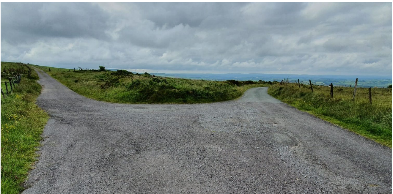
Plate 13-3: Local Road L7461 at Knocknagappul (GCR)
